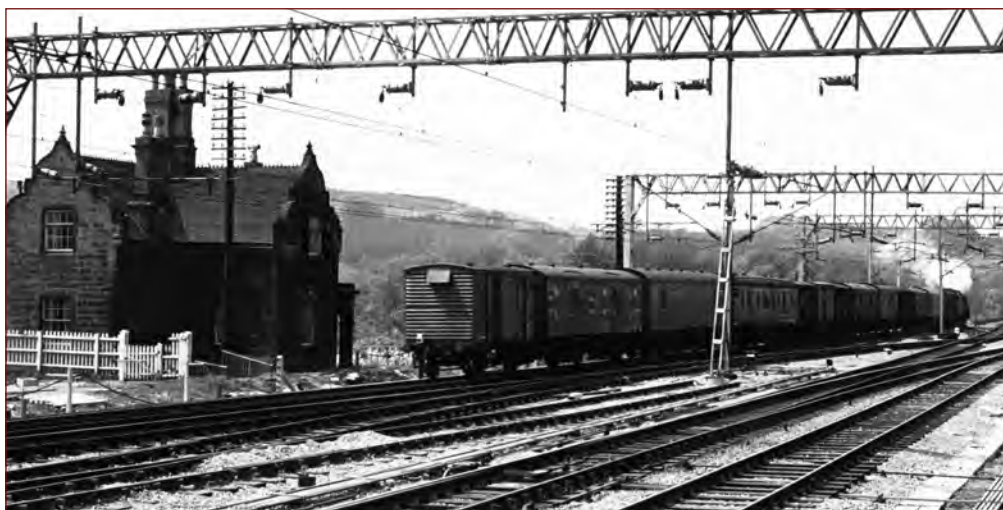
A Down fitted parcels train speeds through the (closed) Colwich station. The building is in the Jacobean style of the North Staffordshire Railway whose Trent Valley line commences here on the right.
