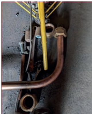
Unions fitted to pick-up pipes (1).
