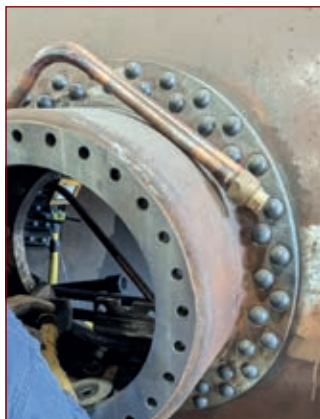
Unions fitted to pick-up pipes (2).
