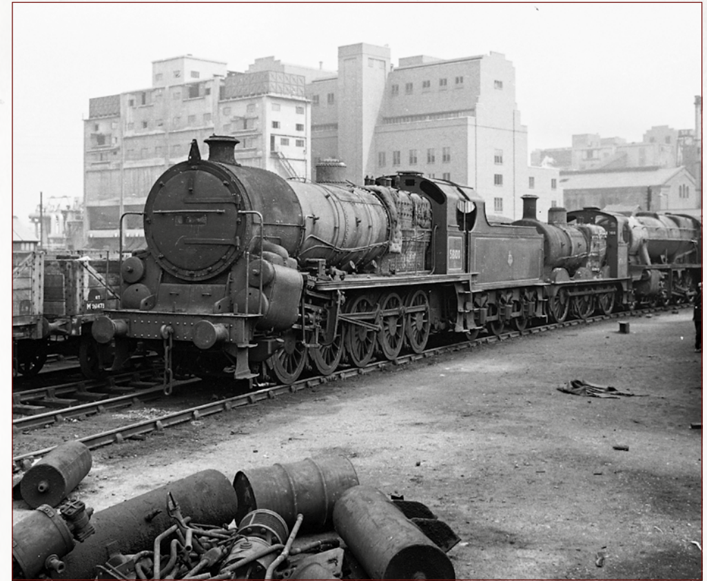
Just over 100 tons of scrap awaiting its destruction which would take place in September 1957. The boiler lagging and front numberplate have been removed whilst the cylinders were supposed to have been removed and saved, intended to show the unusual cross flow arrangement. In the event it is not believed these were retained. The reason No. 58100 remained a one-off was simply that there was no need for further examples; as built it had proved a point that here was a suitable banking engine – also the largest Midland Railway engine ever built. It remains a great pity it was not saved for posterity. © TRANSPORT TREASURY
