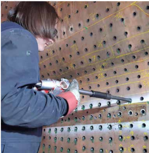
Tapping stay hole in the Inner Firebox.
