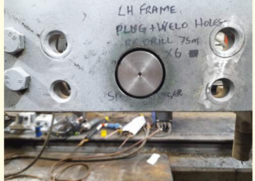
Typical frame repair. Hole re-drilled and plug fitted ready for welding.
