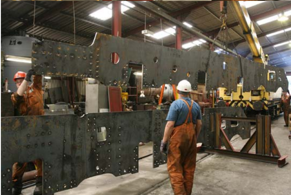
The second frame plate is carefully lowered into position inside the Works.
